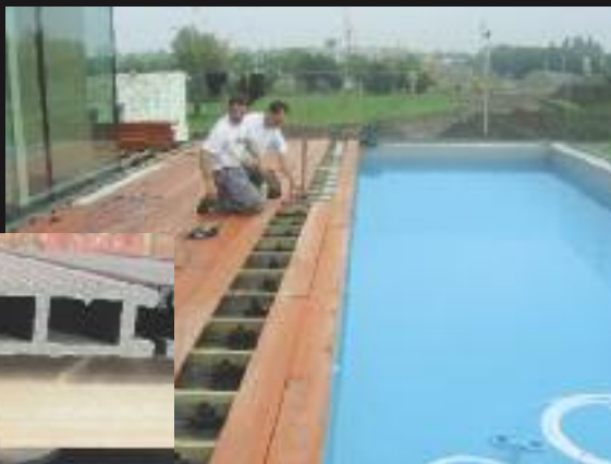
Adjustable support for wooden terraces
