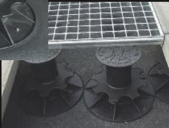
Adjustable support for metal grates
