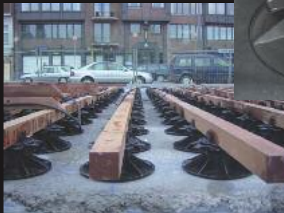
Adjustable support for wooden terraces
